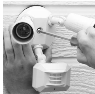
C. Secure base plate to junction box using the Fixture Screw (D). Apply a weatherproof silicone caulk or sealant around the fixture base.
